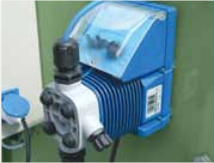
Compound dosing pump
